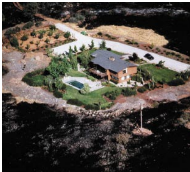
The pre-fire activities implemented by this homeowner included a green and well maintained landscape, reduction of wildland vegetation around the perimeter of the property, a fire resistant roof, and a good access road with a turnaround area. The charred surroundings of the home show that these pre-fire activities effectively protected
